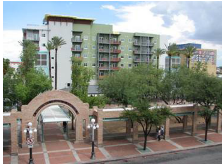
Martin Luther King Apartments, Tucson, AZ
